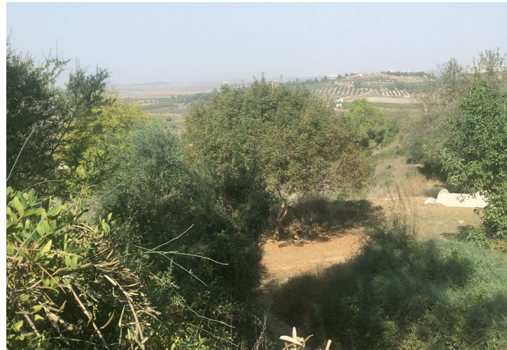
Construction site for the new area of NSWAS.
